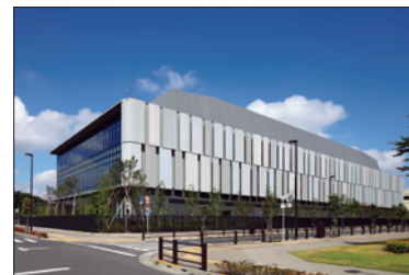
Nishi-Tokyo Data Center
