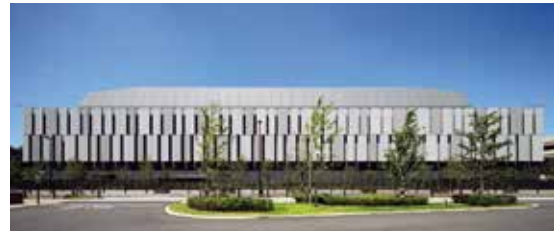
Nishi-Tokyo Data Center
