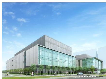
Nishi-Tokyo Data Center
